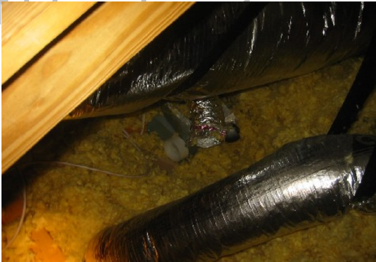
428_Duct disconnected in attic
