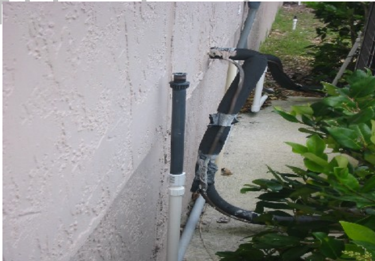
739_Sprinklers installed too close to exterior walls 2
