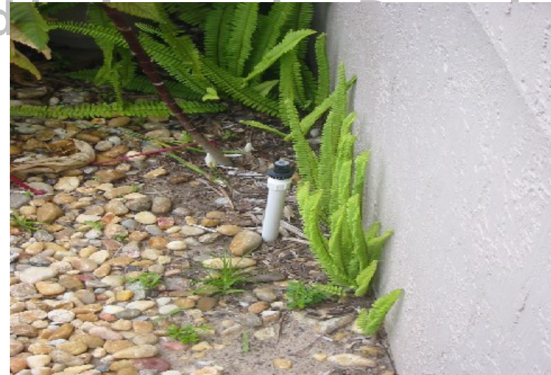
739_Sprinklers installed too close to exterior walls
