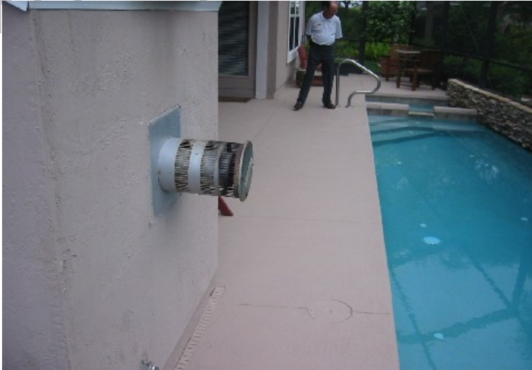
612_Direct vent flue extends too close to pool edge
