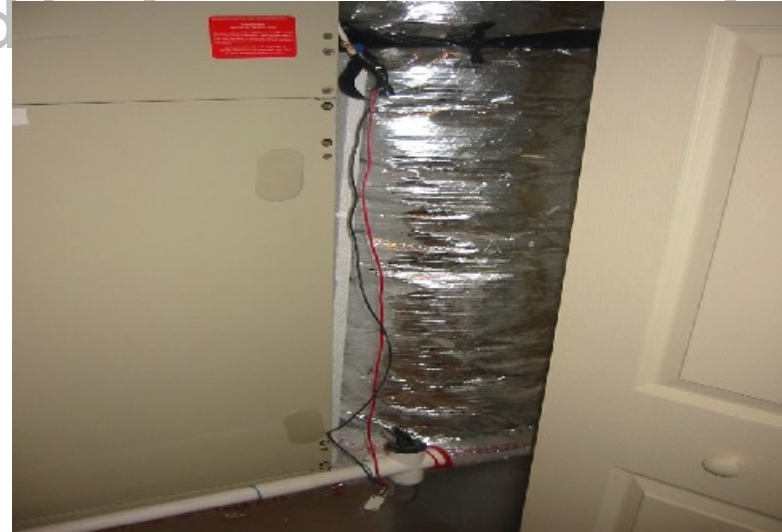
625_Disconnected condensation float
